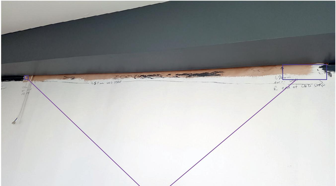
2 x pieces of MDF (or preferred material) to fill in these gaps and be flush with the bottom of the bulkhead.
